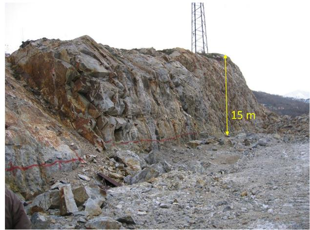
Fig. 4 Slope cut during excavation, showing a horizontal scan-line measurement
