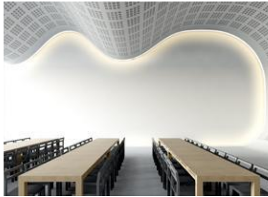
Figure 23 : Plafond Gyptone Curve
