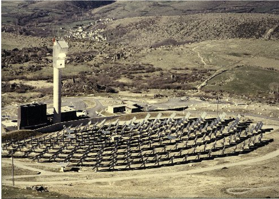
Figure 6 Centrale de Themis (source : google images)
