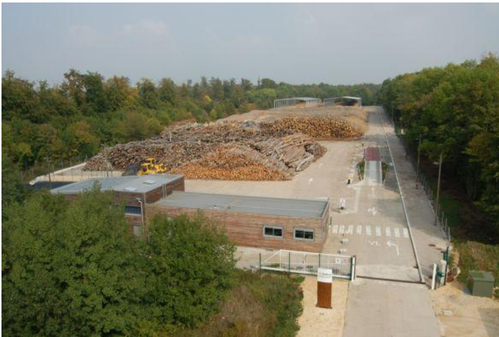
Figure 11 - Plateforme biomasse - Velaine-en-Haye
