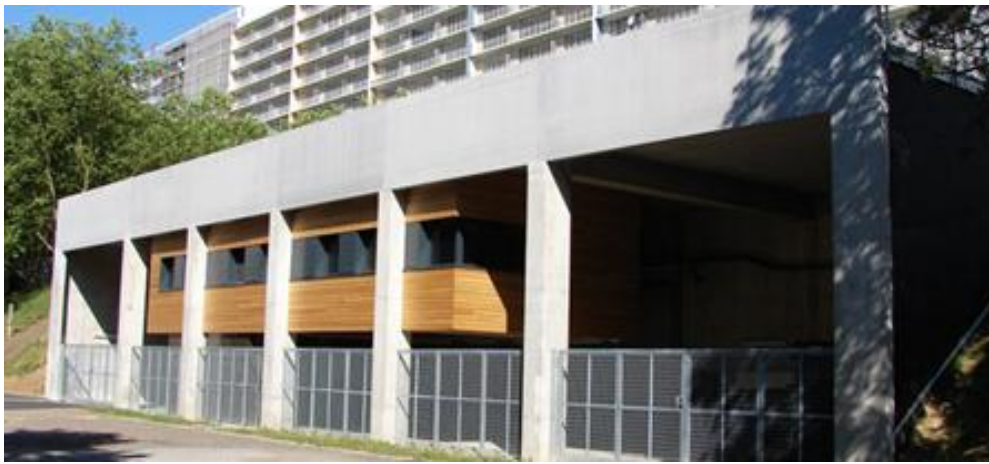
Figure 8 - Chauffage biomasse - Haut-du-Lièvre
