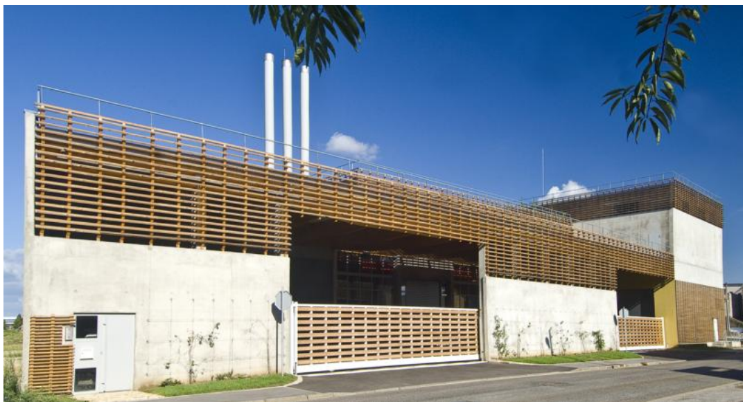
Figure 5 - Chaufferie biomasse Victor
