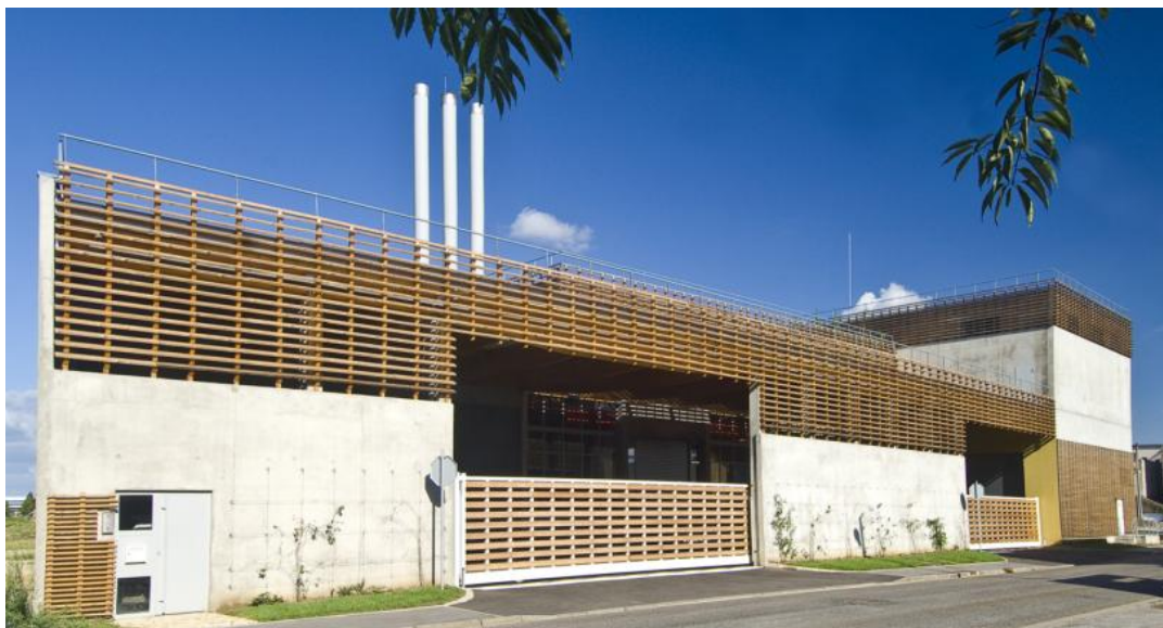
Figure 5 - Chaufferie biomasse Victor
