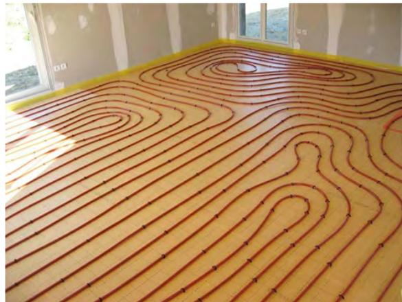
APRÈS DIMENSIONNEMENT :  $L_{\text{PLANCHER CHAUFFANT}} = 250 \text{ M}$
