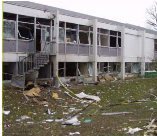
Figure 2 – Example of overpressure damages in the building No 2 located at 50 m in the front of the building No 5, source of the explosion (Neunlist, 2007).
