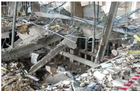
Figure 1: Selection of relevant photographs indicative of the damage on the building No 5 (front of the building – inside laboratory room – collapse of the floor).
