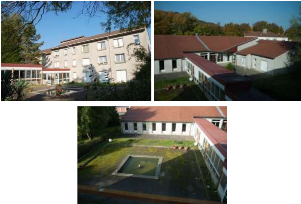
Figure 3 - Photographies de la structure
