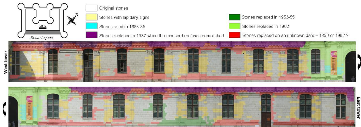
Fig. 4: Distribution of various stone replacements on the south façade
