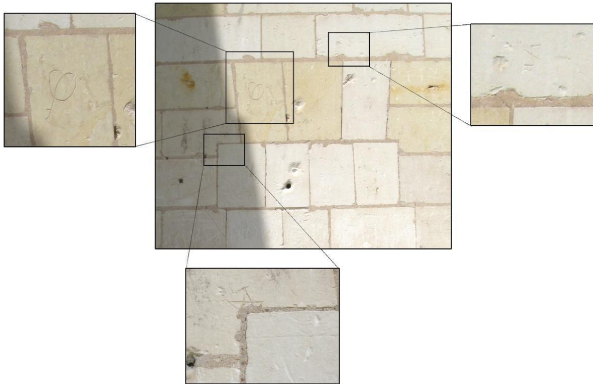
Fig. 2: South façade: door walled on the first left span, with a lapidary sign cut by the addition of a stone to the wall above the door, probably before 1555
