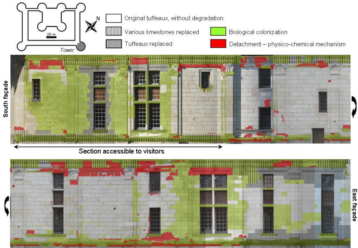
Fig. 7: Age and decay features of stones in the east tower
