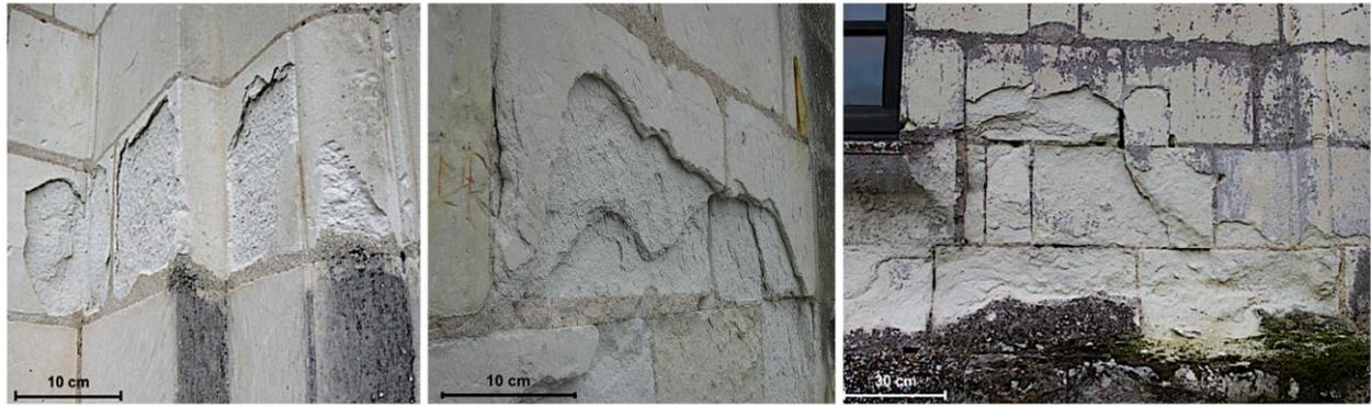
**Figure 1.** Examples of stone spalling at the Castle of Chambord
