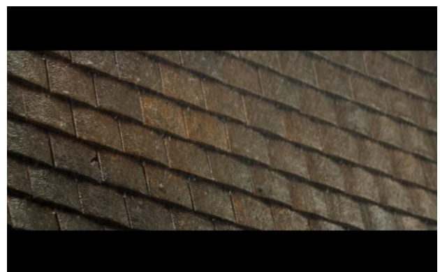
Pattering on the roof (42'51)
