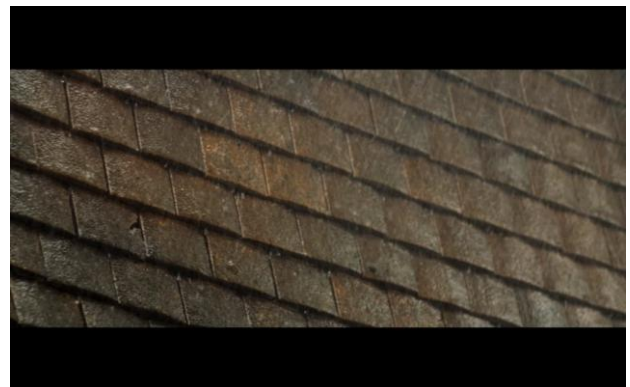
Pattering on the roof (42'51)
