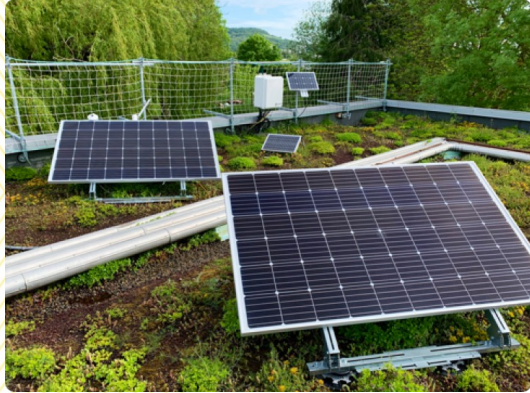
Green roof platform
