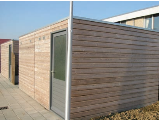
Salvages: Plato®Wood Norway spruce Location: Zuid Beijerland
