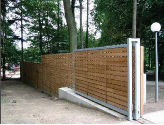
Fencing: Plato® Wood poplar Location: Openlucht Museum, Arnhem
