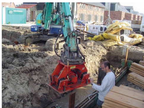
Channel siding: Plato®Wood Norway spruce Location: De Hoorn in Houten
