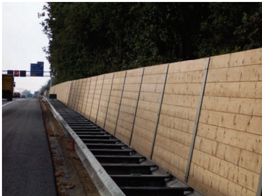
Noise retaining wall: Plato®Wood Norway spruce Location: Sint Joost, A2 (afrit 44)
