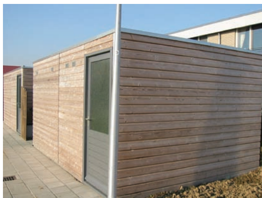
Salvages: Plato®Wood Norway spruce Location: Zuid Beijerland
