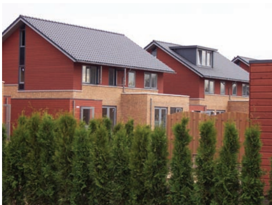
Salvages and cladding: Platomium® Oslo with Olympic Stain Location: Vleuterweide in Vleuten
