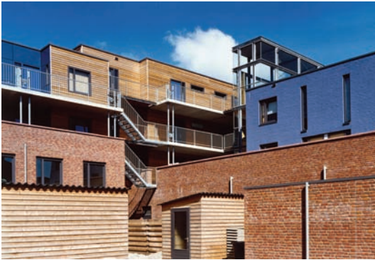
Salvages and cladding: Platomium® Oslo Location: 't Fort, Apeldoorn
