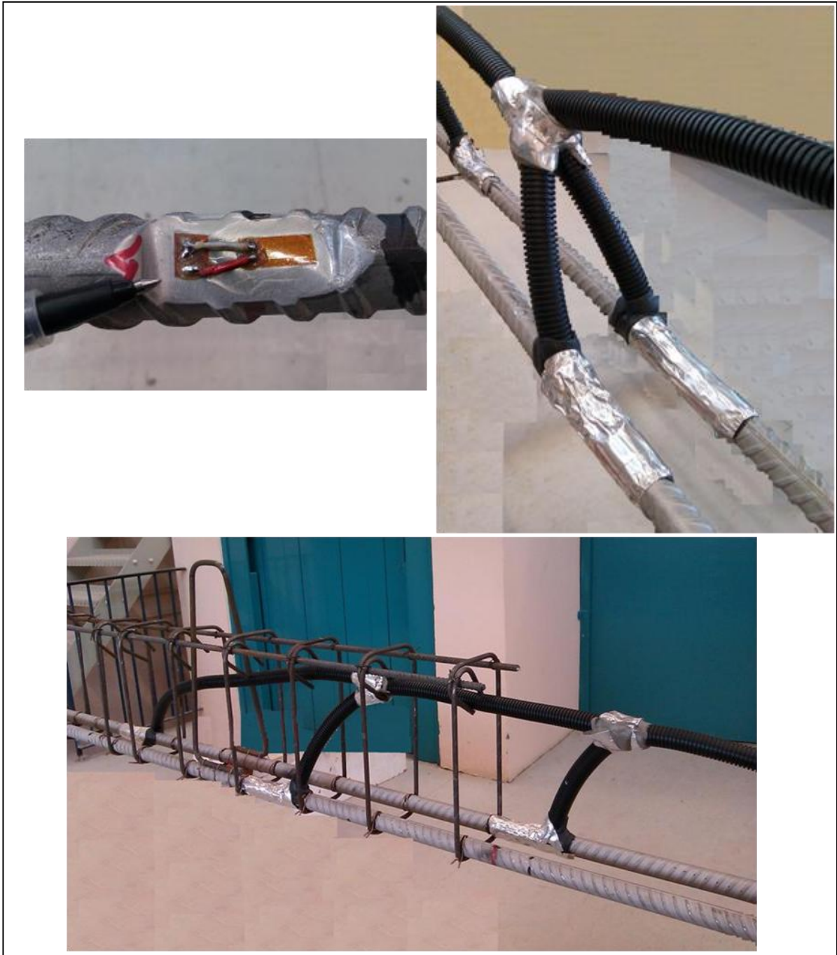
Fig. 3.17. Strain gauges on the reinforcing bars
