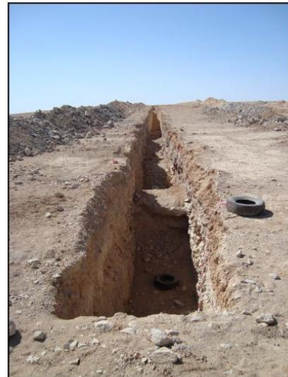
Figure V. 3. Trench T07 (L:200m, w:1.5, d:3m)
