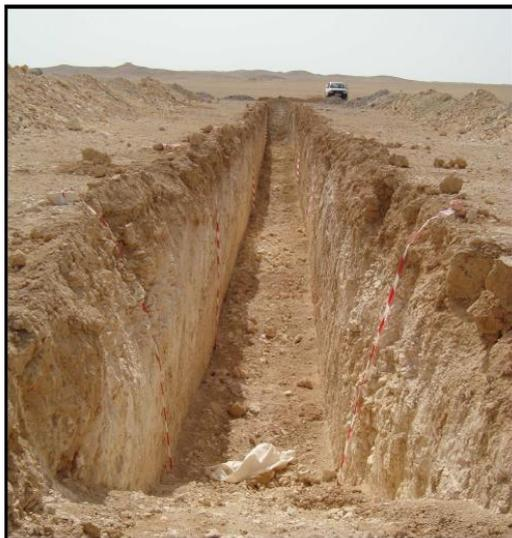
Figure V. 2. Trench T21 (L:200m, w:1.5, d:3m)
