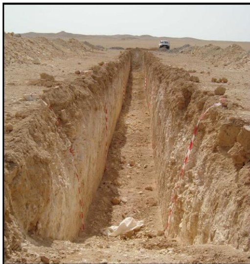
Figure V. 2. Trench T21 (L:200m, w:1.5, d:3m)
