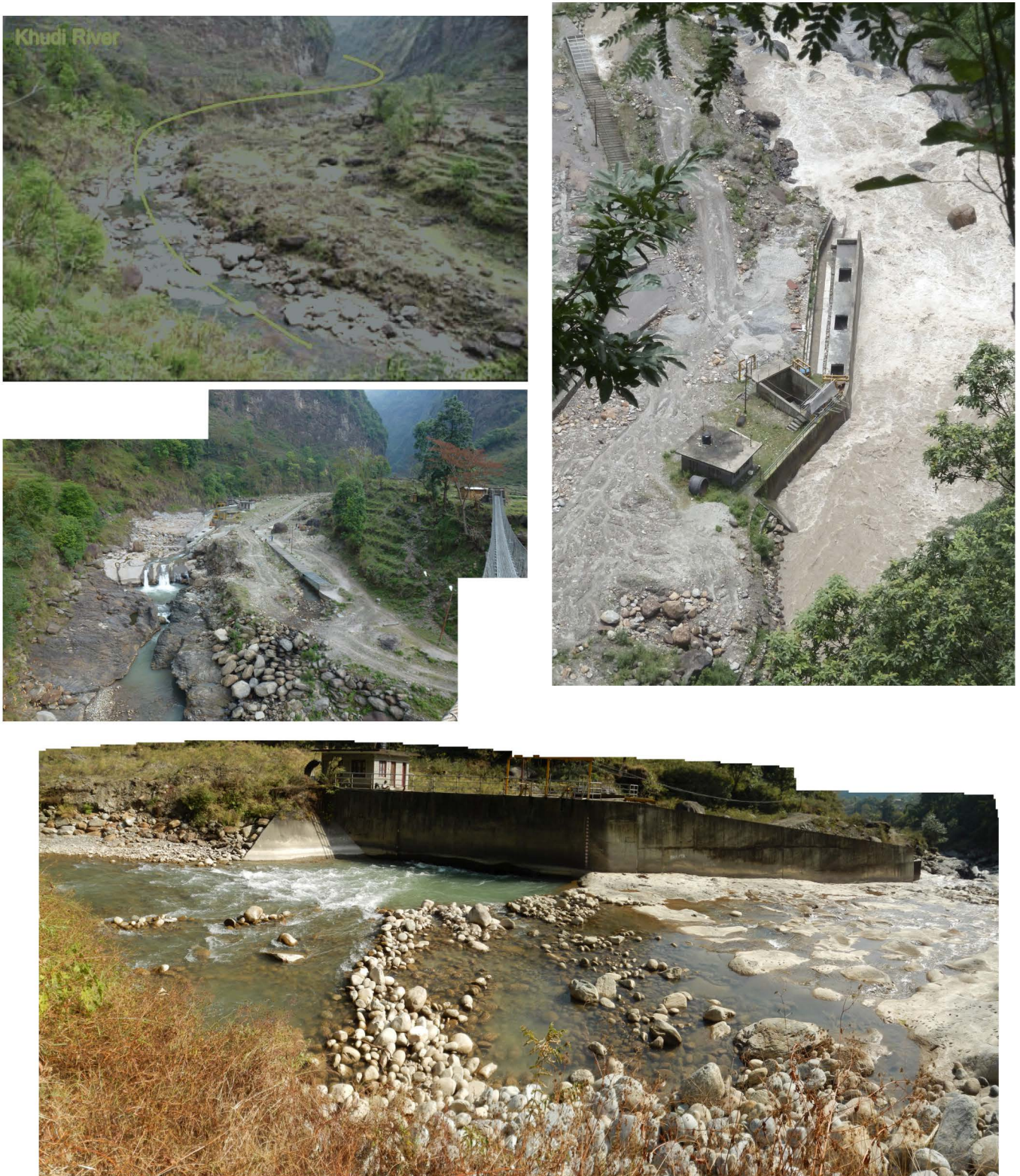
Figure B1: Intake setting constituted by a vertical wall on the Khudi left bank, a concrete weir and ramp and a boulder evacuation channel down to the base of the ramp. Top left pictures were taken from below the structure and offer a view on the Khudi river before (Shrestha and Phuyal, 2006) and after intake dam completion. The
