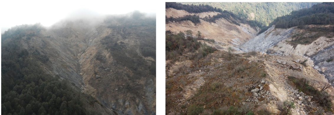
Figure 2 - Pictures from the landslide, from the lower part, looking to SSW (left) and from the northern flank of the active zone, looking to NNE (right)
