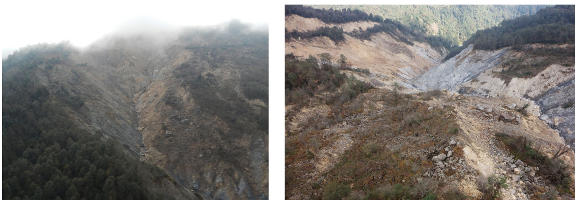
Figure 2 - Pictures from the landslide, from the lower part, looking to SSW (left) and from the northern flank of the active zone, looking to NNE (right)
