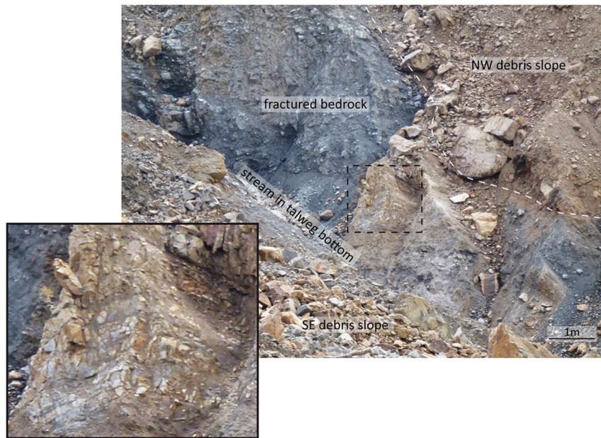
Fig. 3. Bedrock at the scar bottom in the southern branch of the Saituti landslide (see location in Fig. 2) displaying intense fracturation.
