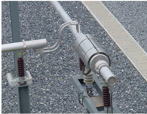
a) DC measuring devices
