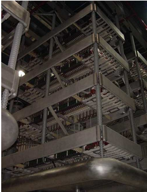
b) Valve tower
