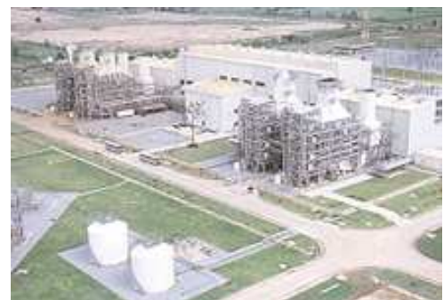
e) 2024 MW, Wang Noi Power plant, Ayutthaya province
