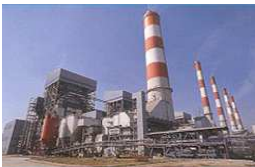
b) 2625 MW, Mae Moh Power Plant, Lampang province
