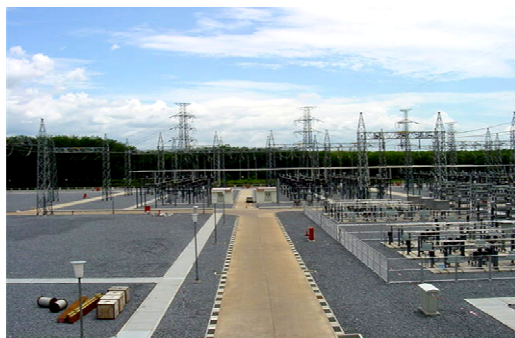
b) Relay house
