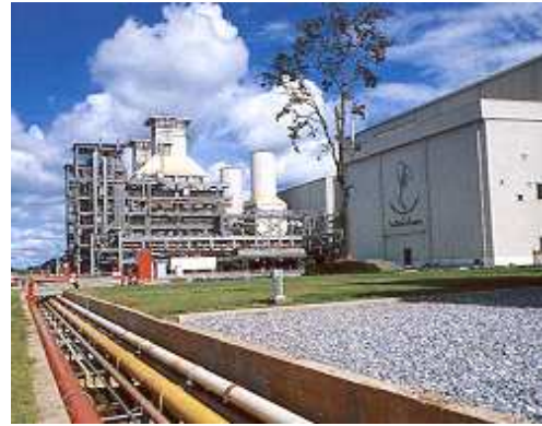
d) 710 MW, Nam Phong Power Plant, Khon Kaen province
