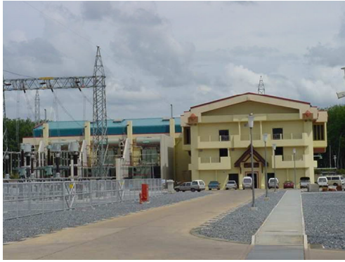
a) Converter building
