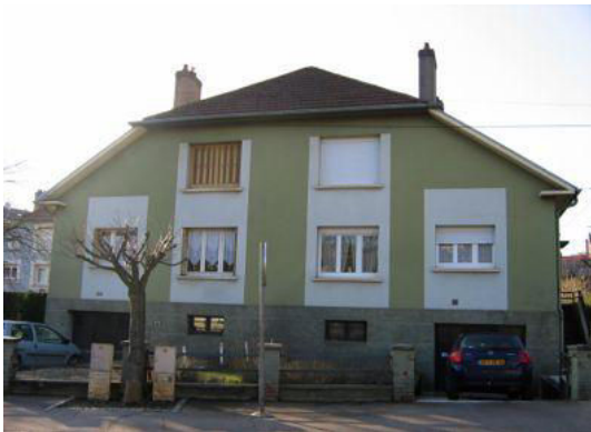
Building No.486 in zone 9
