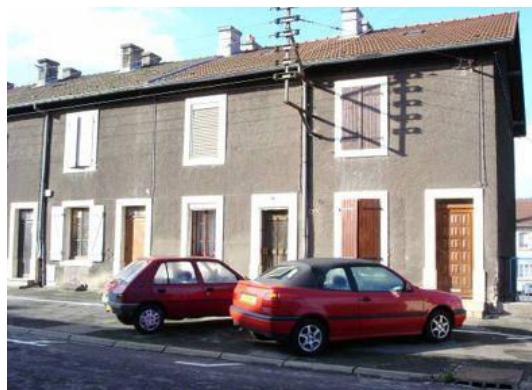
Building No.14 in zone 10
