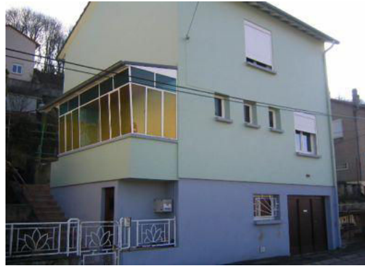
Building No.145 in zone 2C
