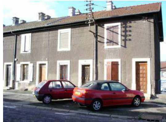
Unreinforced masonry building in zone 10
