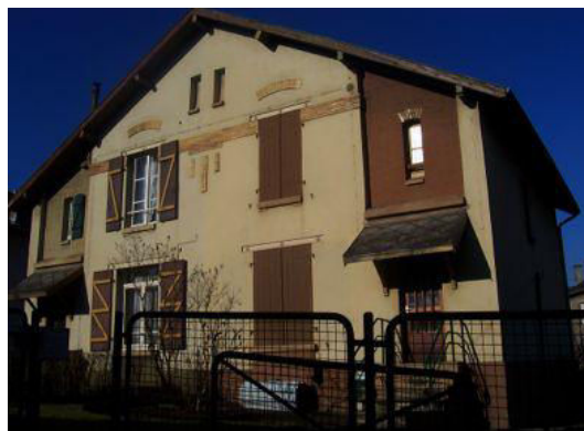
Building No.208 (Parcelle 177-178) in zone 6A
