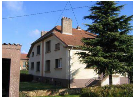
Building No.14 in zone 9
