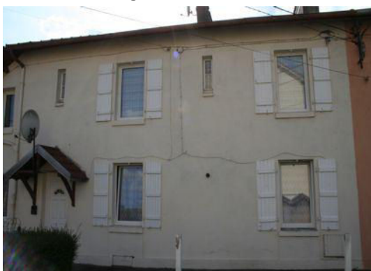
Building in zone 11
