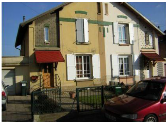
Building No.1000 (Parcelle 249-250) in zone 5A
