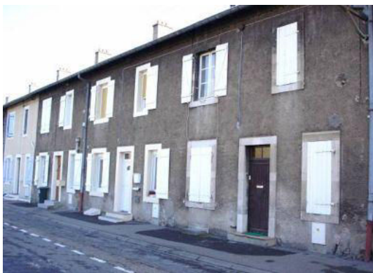
Building No.1436 in zone 10
