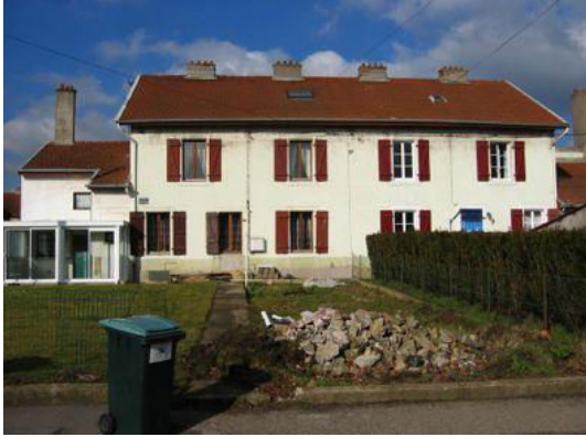
Unreinforced masonry building in zone 1
