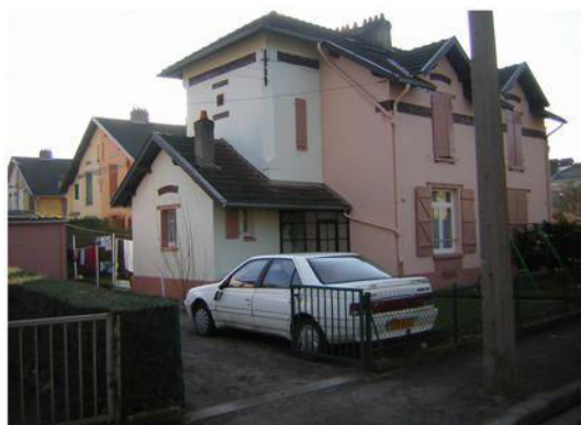
Building No.994 (Parcelle 174-175) in zone 5B
