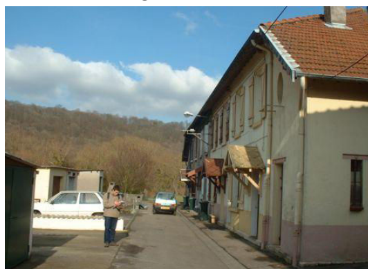
Building No.898 in zone 10
