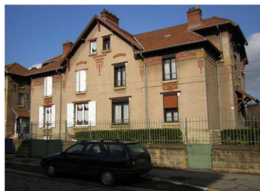
Building No.963 (Parcelle 216-217) in zone 5E
