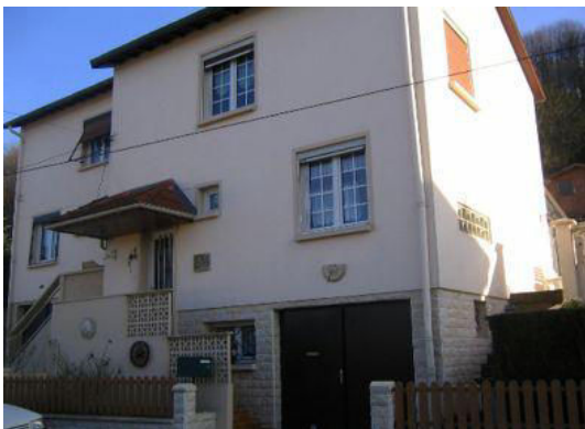
Building No.140 in zone 2B
