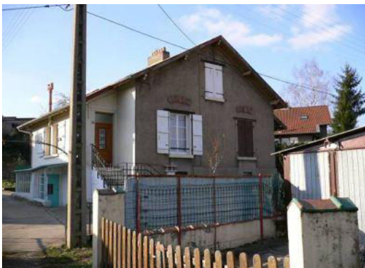
Building No.330 (Parcelle 112) in zone 3
