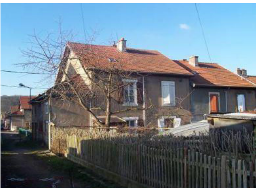
Building No.1121 (Parcelle 1350-1351) in zone 7
