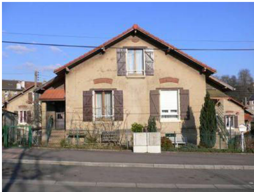
Unreinforced masonry building in zone 3
