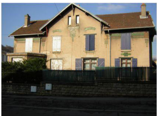
Building No.1004 (Parcelle 245-246) in zone 5E
