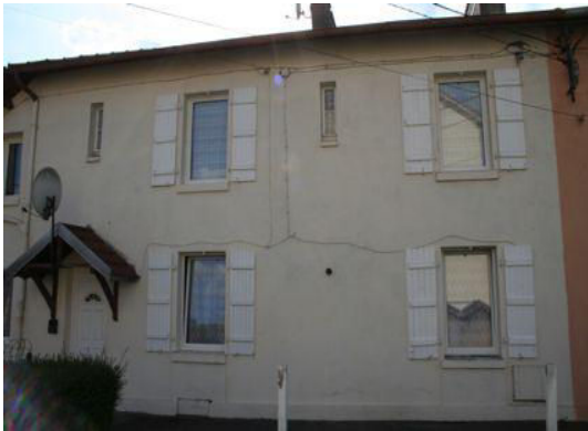
Building in zone 11
