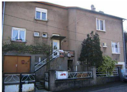
Building No.131 in zone 2B
