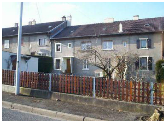
Building No.1259 (Parcelle 1422-1425) in zone 7
