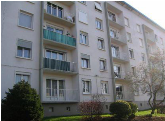
Building No.167 in zone 2D
