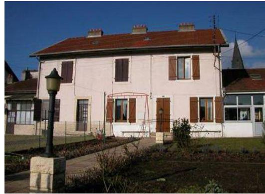
Building No.692 (Parcelle 372-373) in zone 1
