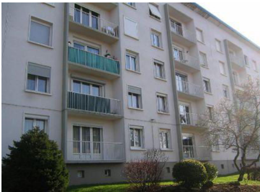
Building No.167 in zone 2D
