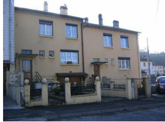
Reinforced masonry building in zone 2
