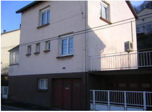
Building No.143 in zone 2C
