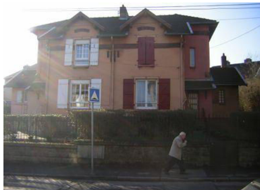
Building No.1036 in zone 6B
