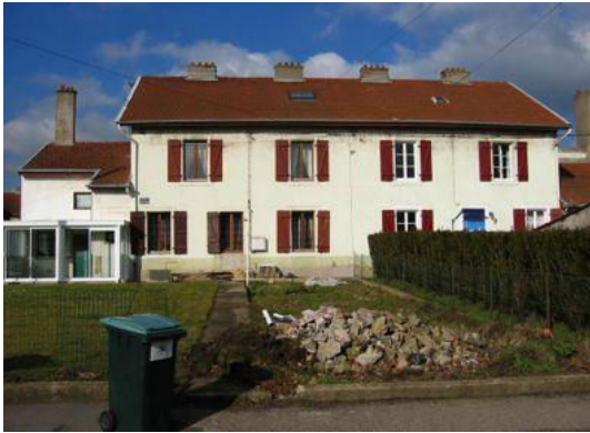
Building No.50 (Parcelle 648) in zone 1
