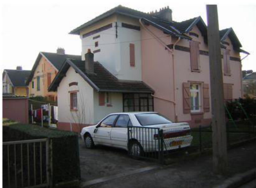
Building No.994 (Parcelle 174-175) in zone 5B
