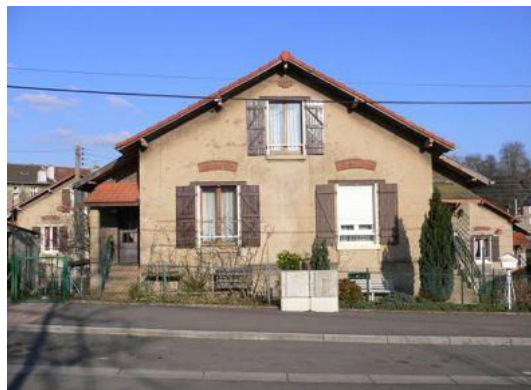
Building No.334 (Parcelle 89) in zone 3
