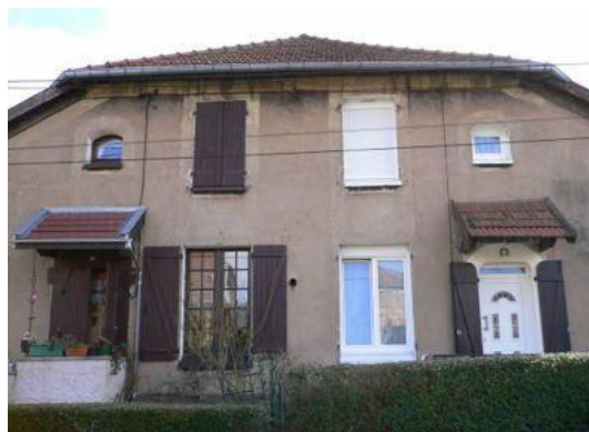
Building No.549 (Parcelle 660) in zone 4
