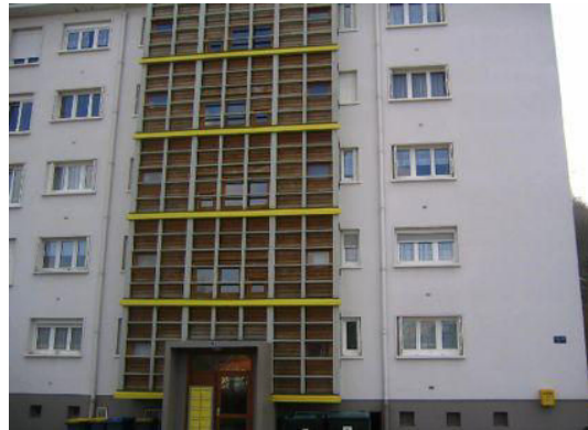
Building No.218 in zone 2D
