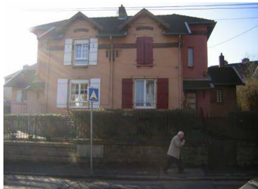
Building No.1036 in zone 6B
