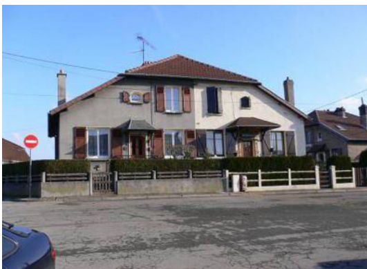
Building No.525 (Parcelle 676) in zone 4
