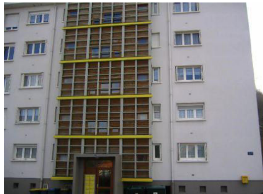
Building No.218 in zone 2D
