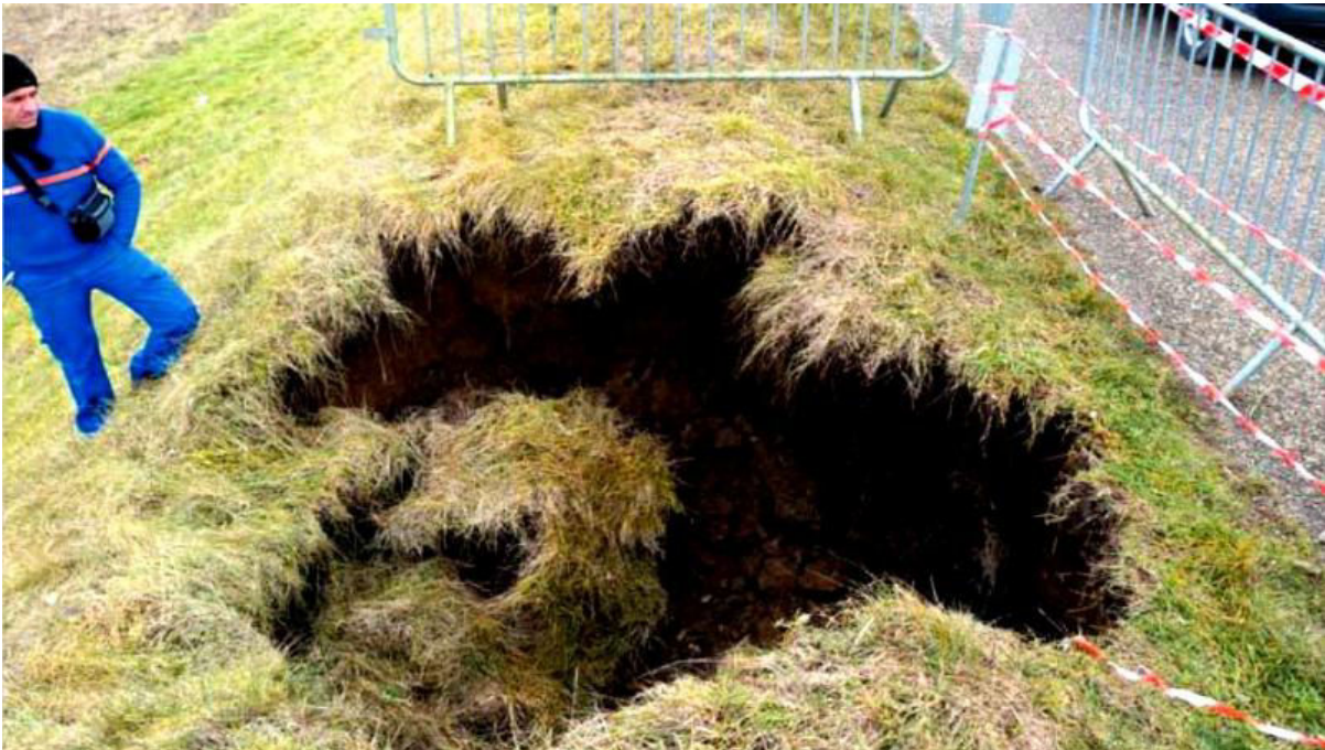
Figure 99 Sinkhole on the head of the dike of Val d'Orléans in area of Jargeau (Dore and Mathon 2011).
