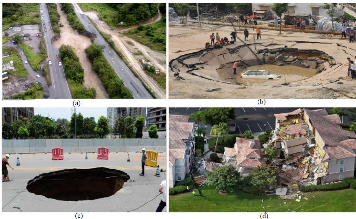
Figure 5 Effect of karst sinkholes on several civil structures. (a) An aerial view of the damaged a highway in the State of Miranda (Venezuela) 2010 (Photo by Miranda Government/Reuters), (b) A collapsed road surface in Guangzhou, Guangdong Province (China) 2008 (Photo by Reuters/China Daily), (c) Sinkhole in the main road in Changsha (China), 2012 (photo by Quirky China News / Rex Features), and (d) Buildings collapse into a sinkhole, Clermont, Florida, USA 2013 (photo by Red Huber/Orlando Sentinel/MCT).
