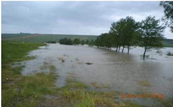
Fig. 6.57 Ezer Pond – dam’s body –flooded downstream bench
