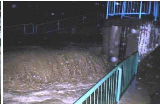
Discharge blade from downstream toward upstream
