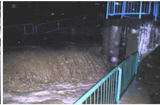
Discharge blade from downstream toward upstream
