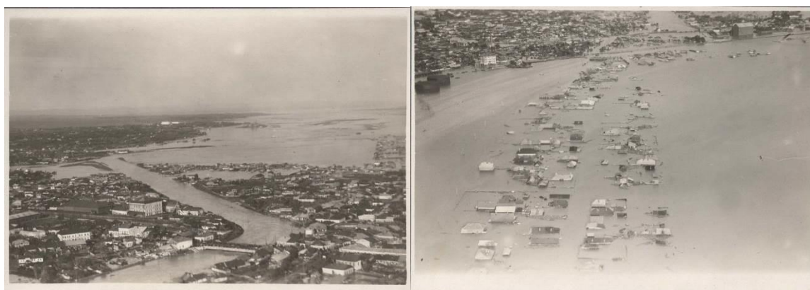
Fig. 6.33 Inundations in Iași, 1932 (National Archives photos)
