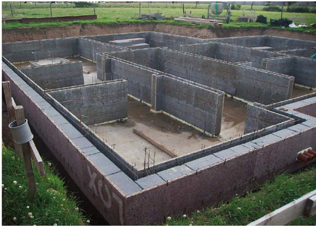
Fig. 1. Wood cement panels as permanent formwork.
