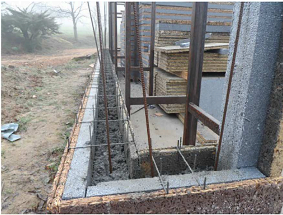
Fig. 1. Wood cement panels as permanent formwork.
