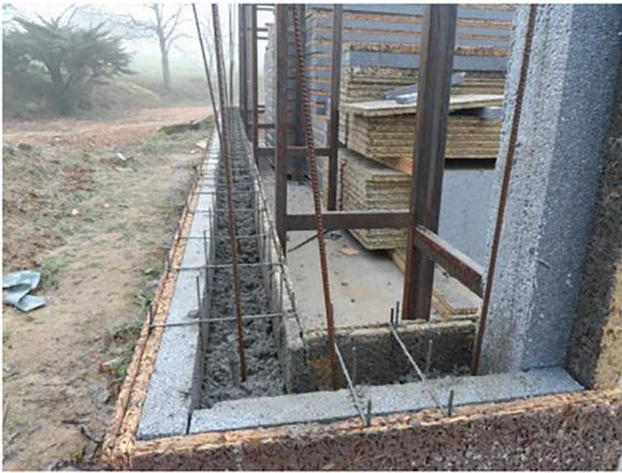
Fig. 1. Wood cement panels as permanent formwork.
