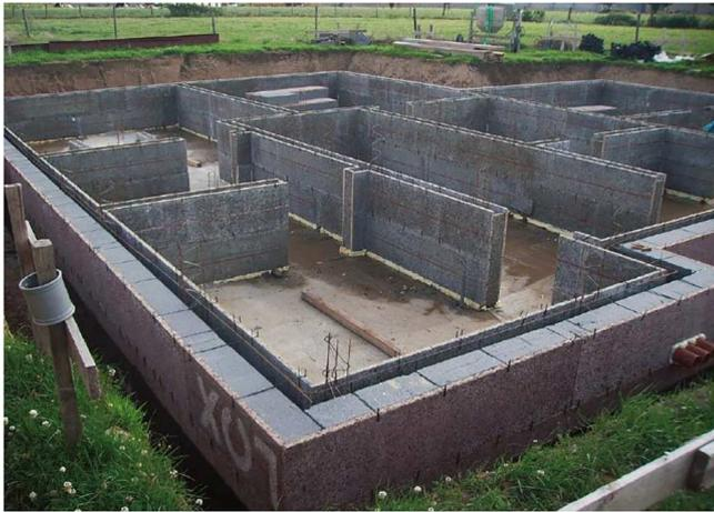
Fig. 1. Wood cement panels as permanent formwork.
