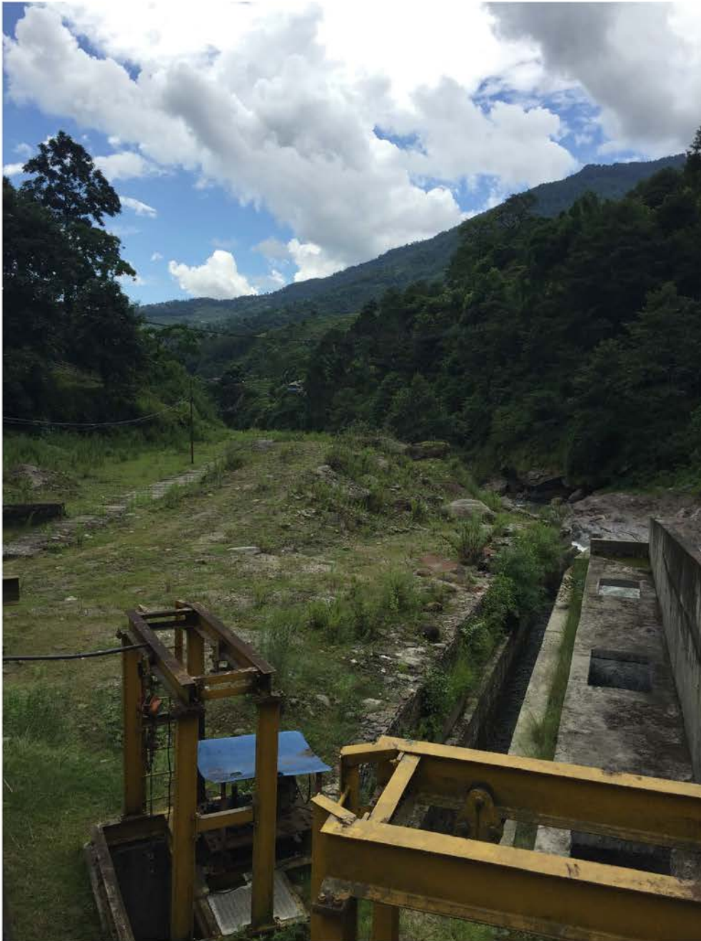
Figure 2.12 – A view of the water station at the hydro-electric power plant located approximately 4.5 km upstream from the Khudi’s confluence with the Marsyandi. This is the location of the hourly water sampling that was completed in 2013 and 2015 (see Chapter 4). The long drainage system is the entry point for water from the Khudi to enter into the hydro-electric power plant.
