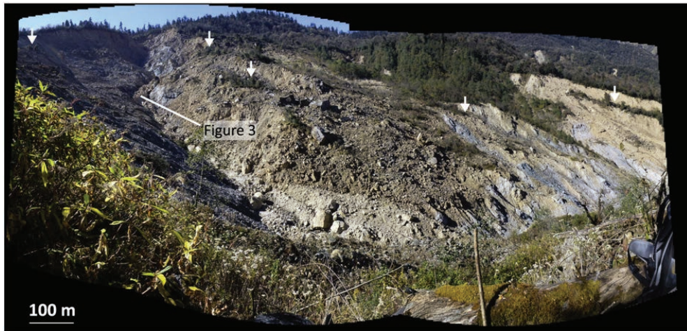
Figure 2.11 – View of the Saituti landslide from Gallo and Lavé (2014)
