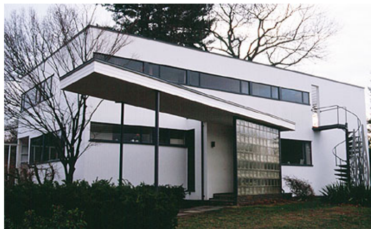
Figure 53: Maison de Walter Gropius, 68 Baker Bridge Road Lincoln, Massachusetts 01773USA. 161
