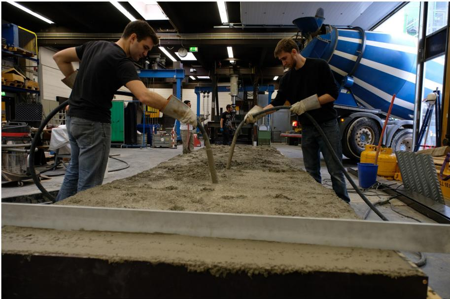
**Figure 6.14** – Concrete vibrated
