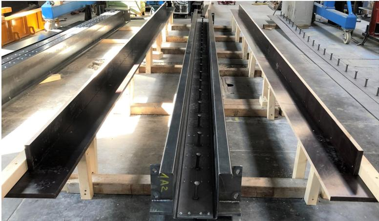
Figure 6.3 – The steel beam placed in the formwork
