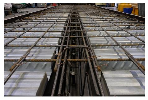
Figure 6.10 – The stirrups linked to the reinforcing mesh
