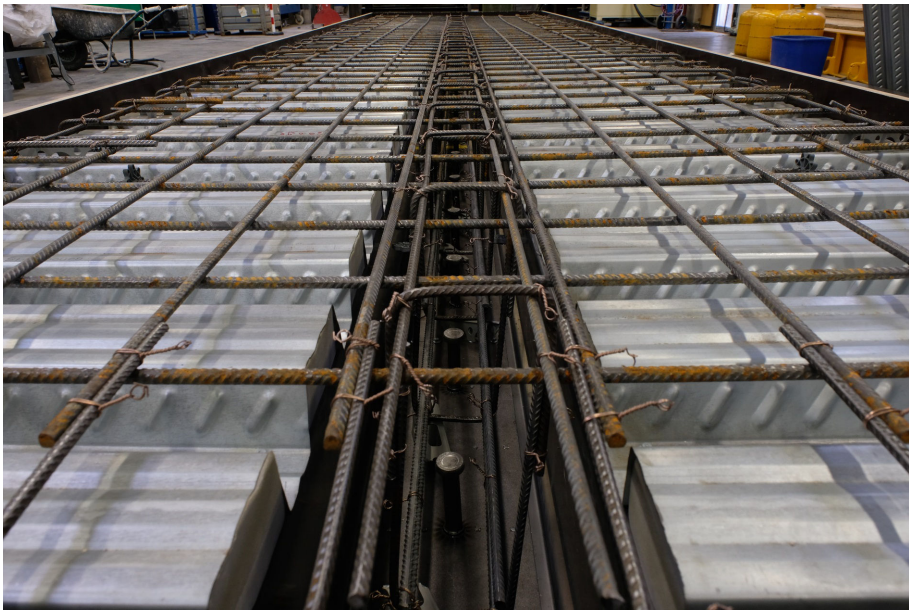
Figure 6.10 – The stirrups linked to the reinforcing mesh
