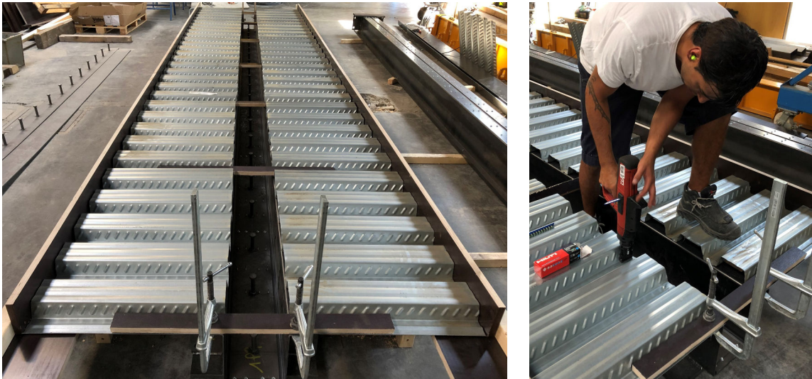
(a) Positioning of the steel decks
