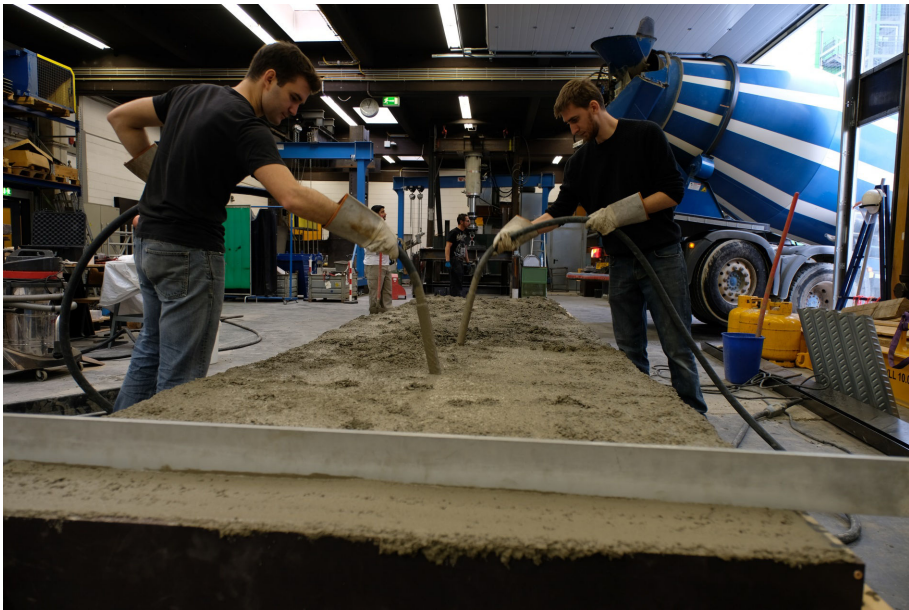
Figure 6.14 – Concrete vibrated
