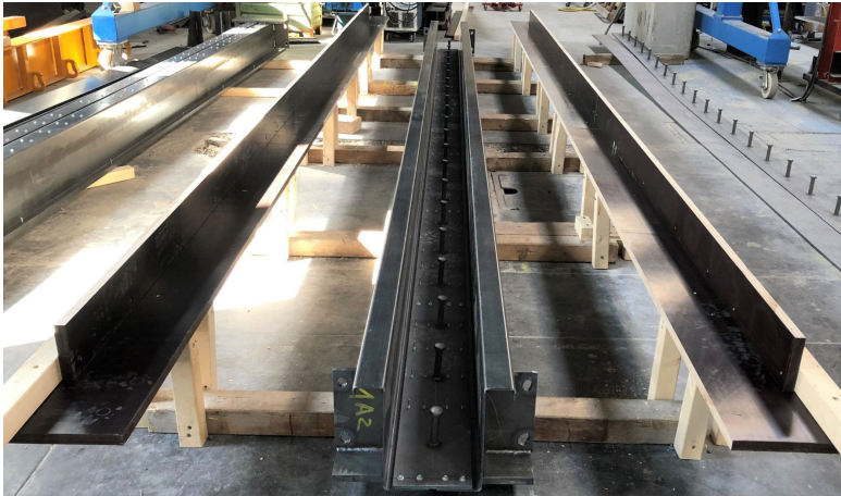
Figure 6.3 – The steel beam placed in the formwork
