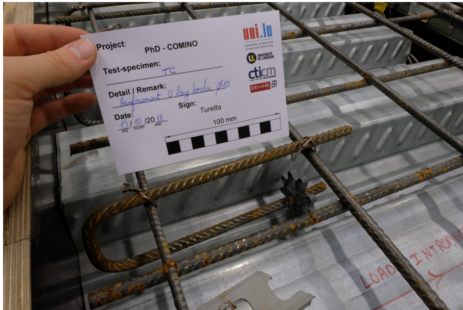
Figure 6.12 – Rebars folded in U at the edge of the composite slab (HA10)
