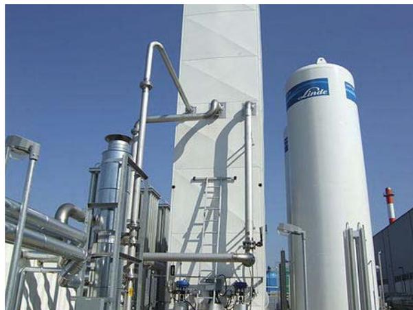
*Figure 1.1: Cryogenic distillation industrial plant (Linde company)*
