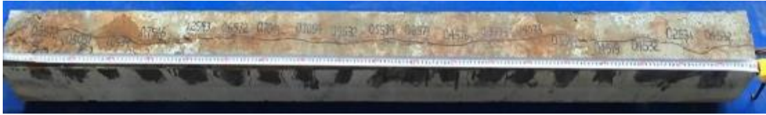
Fig. 3.6. Longitudinal crack of specimen
