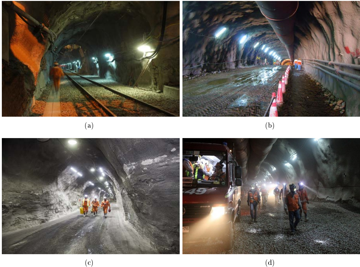
Figure 3.4: El Teniente underground mine light deployment (a) Transportation tunnel (b) Machinery working inside the tunnel(images by Codelco)
