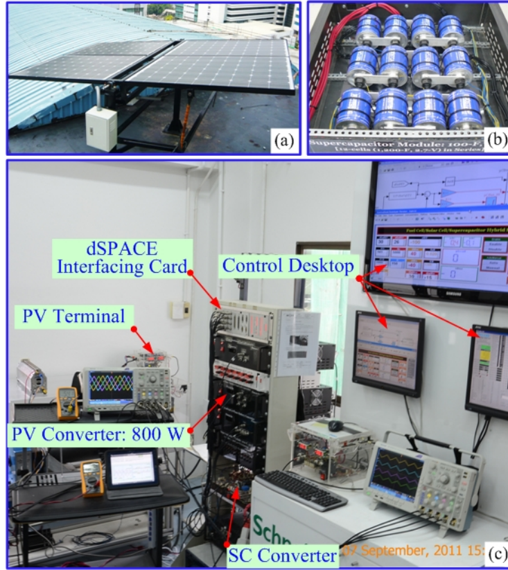
Fig. II.3.59. Photograph of a test bench power plant. (a) solar cell panels, (b) SC bank, and (c) test bench.
