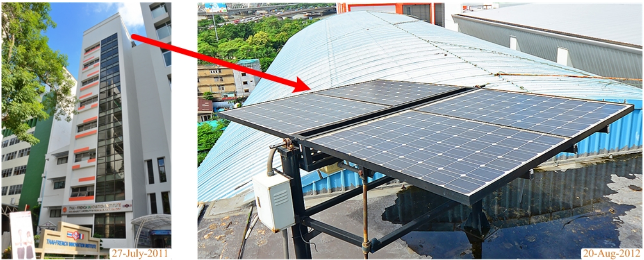
Fig. II.2.23. PV panel (Ekarat Solar, 800 W) is installed on the roof of the laboratory building (KMUTNB, Thailand).
