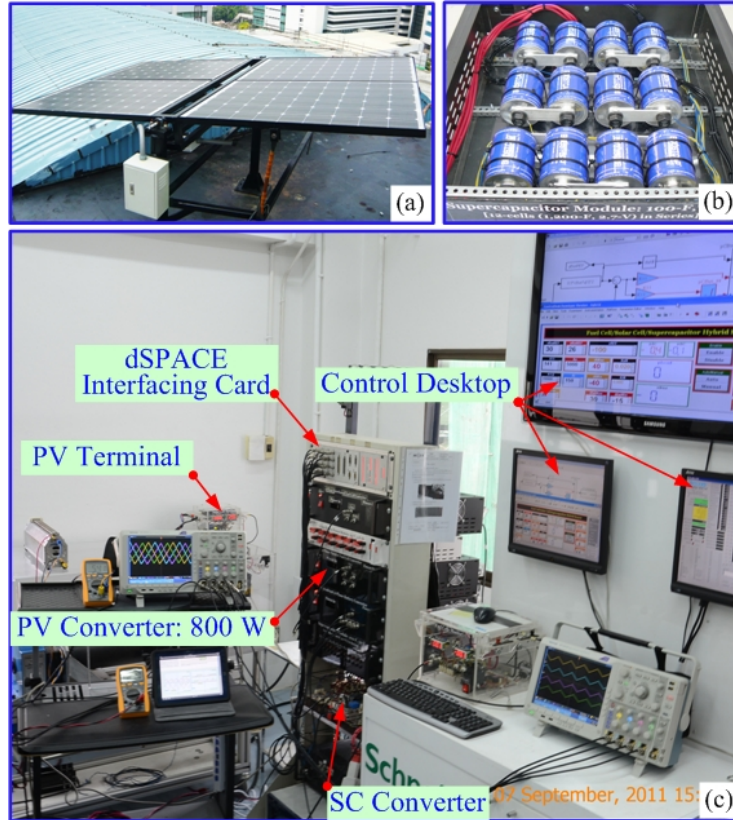
Fig. II.3.59. Photograph of a test bench power plant. (a) solar cell panels, (b) SC bank, and (c) test bench.
