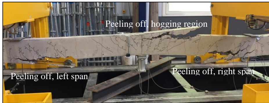
Figure 2-13 : Failure mode of beam BC3-L
