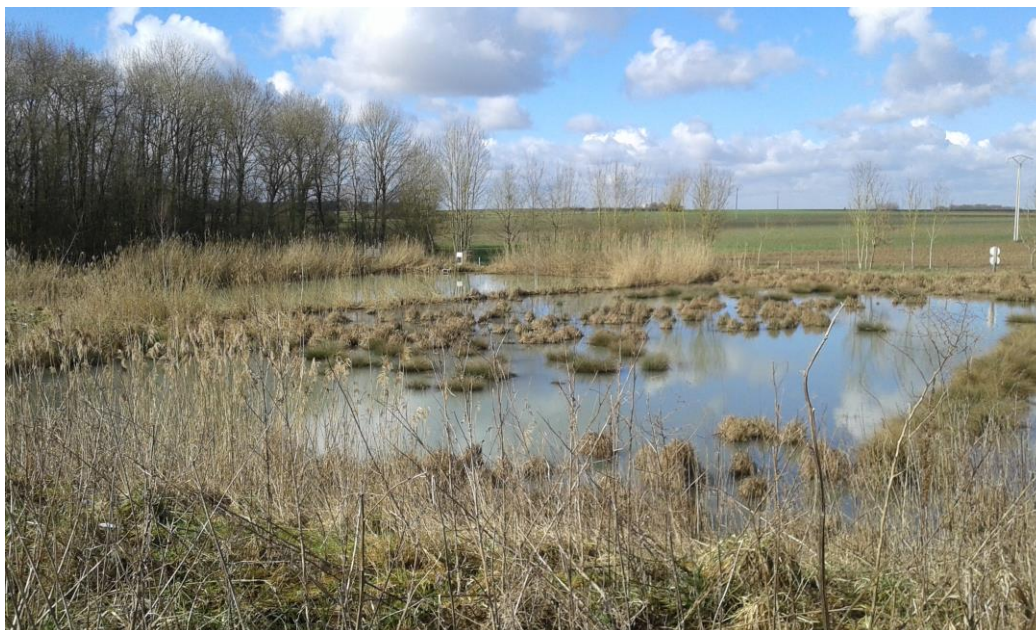
Photo 3.1. The constructed wetland in Rampillon (Seine et Marne, FR) (Photo by Author).
