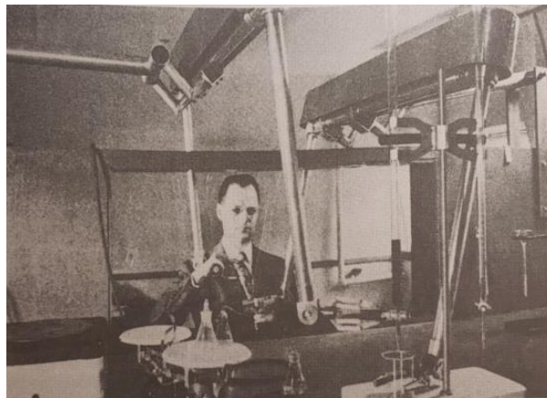
Figure 1.2 First mechanical telemanipulation system
