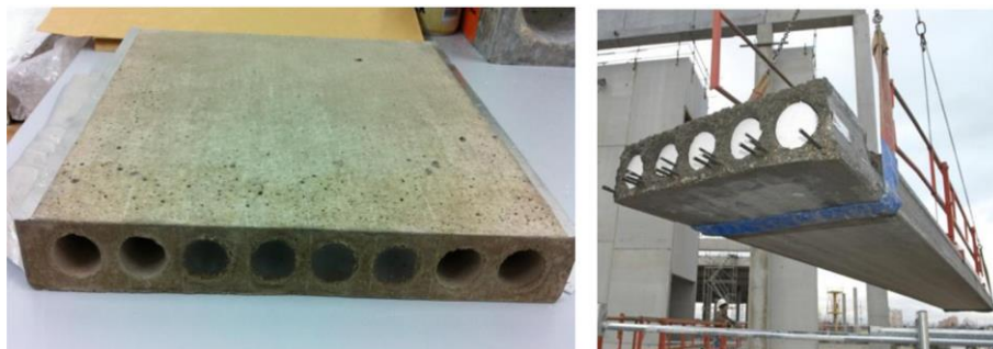
Fig. 2.11. Floor panel incorporated with PCM [142]
