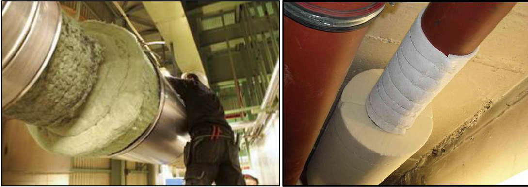
Figure 4.5. Common insulation of industrial pipes (left). Thickness comparison between normal insulation (lower part), aerogel-based insulation (Aspen Aerogel) (middle part) and row pipe (upper part) (right).
