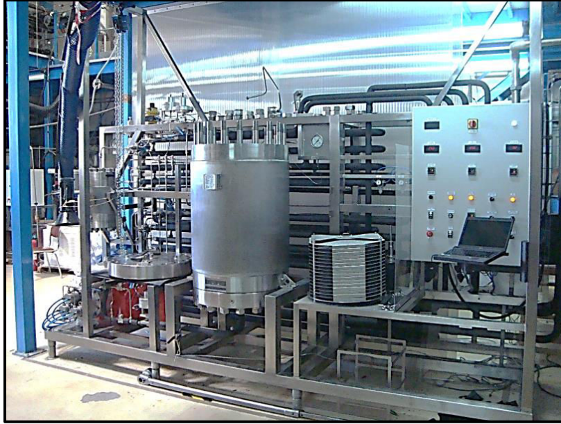
Figure 3.3. Final assembly of the plant.
