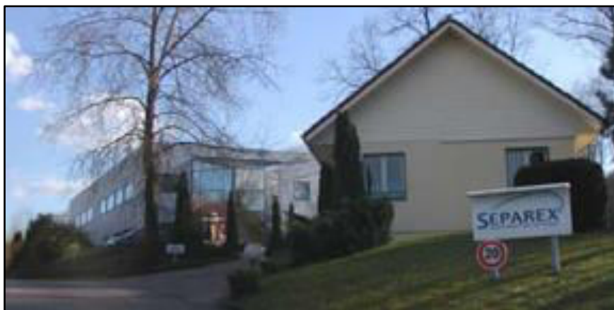
Figure 4.1. SEPREX S.A.S. Facilities in Champigneulle France.
