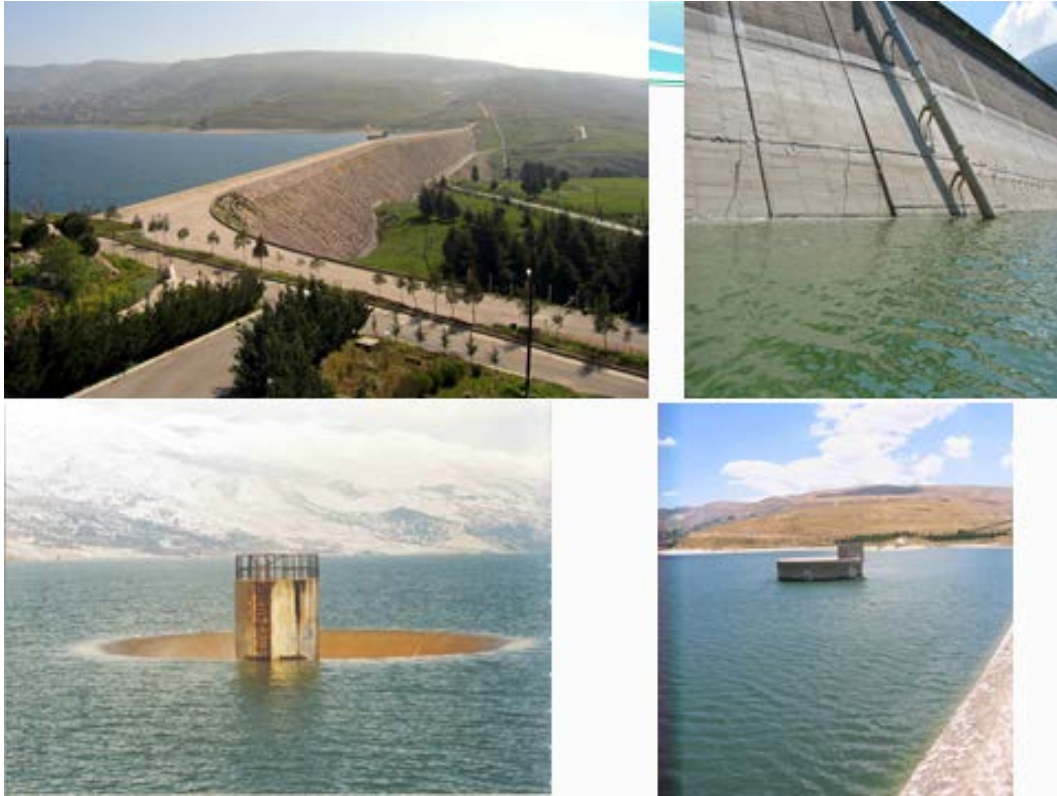
Figure 18: Litani hydro power plant (by litany.gov.lb)
