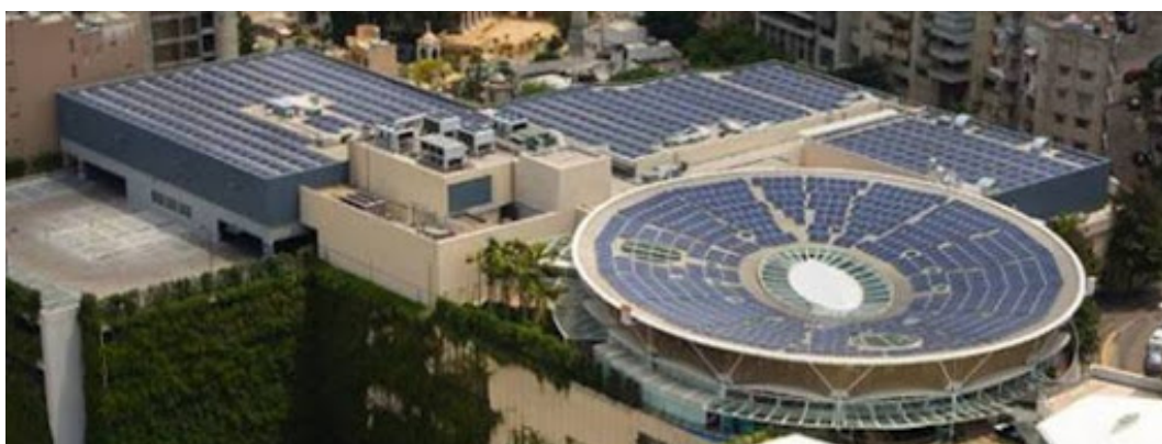
Figure 21: One of the Largest Private installed PV Plant in Lebanon (ABC Achrafieh)
