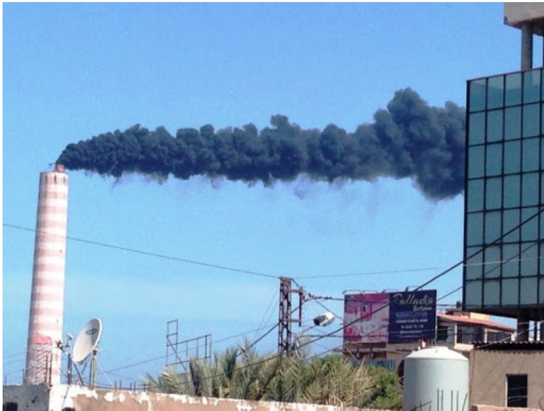
Figure 10: Thermal power plant in Lebanon (Al- Zawq)
