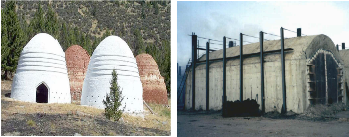
Figure 23. (a) Honeycomb kilns and (b) Missouri kilns [87]
